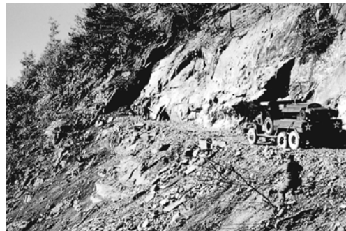
Blasting a road through the mountains for defense on the 38 th Parallel
