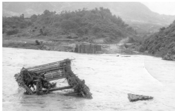
Remains of a 490 ft. Bailey Bridge our unit put across the Han Tan River near Chorwan, Korea. (August, 1952)
